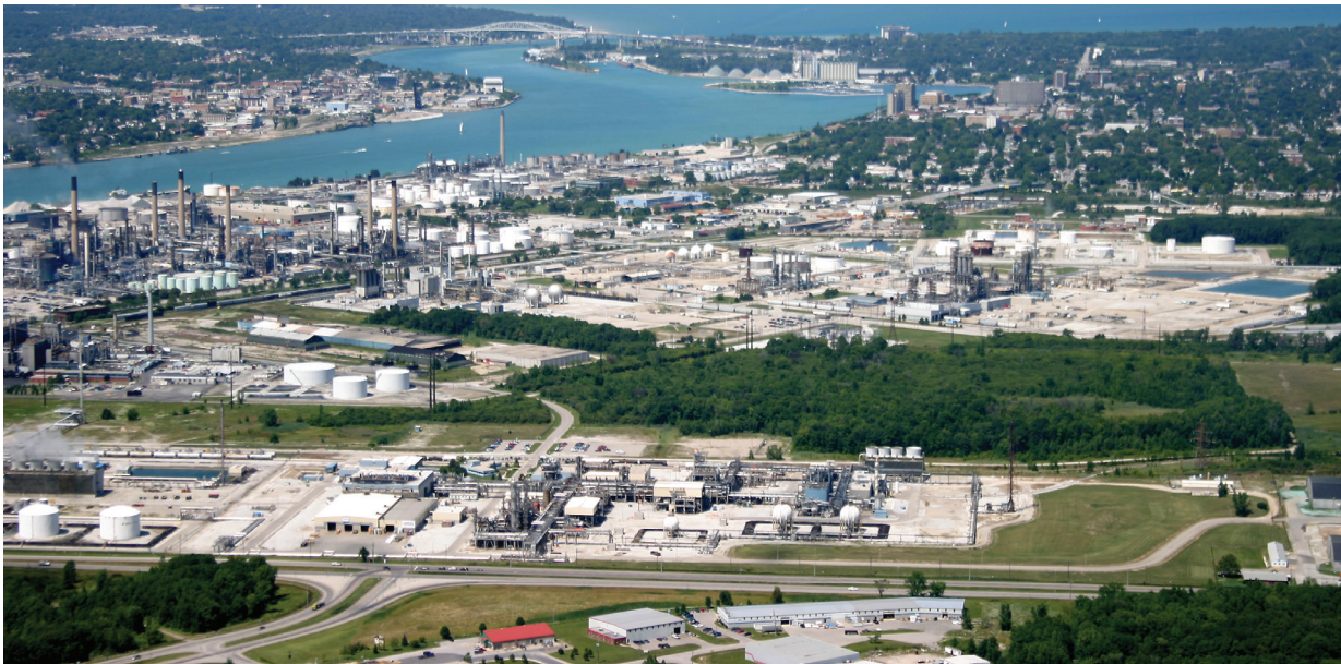
Imperial's Sarnia operation is our most integrated fuels, chemicals, manufacturing and petroleum research facility in Canada. The refinery can process 120,000 barrels of crude daily.
