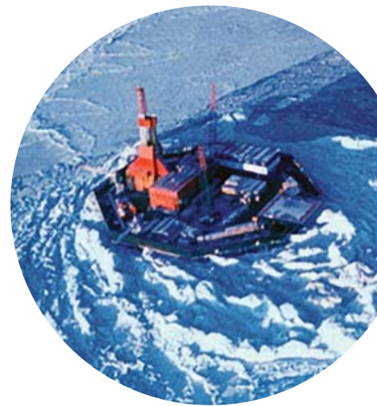
Beaufort Caisson Retained Island (CRI)
