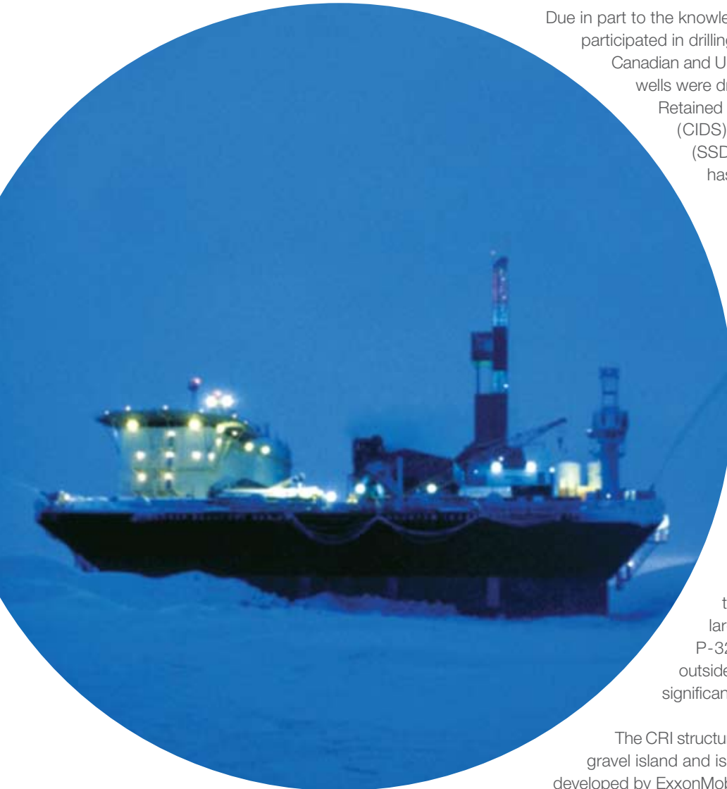
Concrete Island Drilling System (CIDS) at Antares
