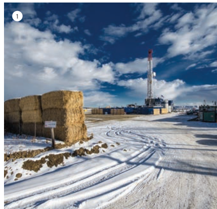
1. Straw bales act as sound barriers during drilling and completion phases for tight oil operations in Alberta. 2. In northeastern British Columbia, directional drilling techniques reduce the surface footprint of operations.
