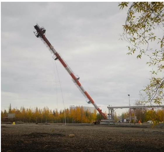
Flare stack removal video
