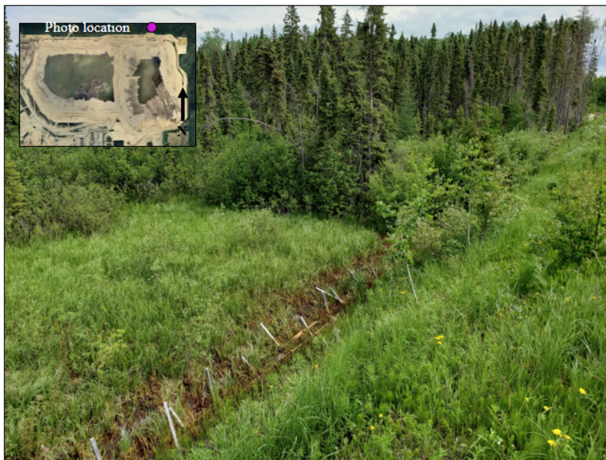
Figure 1.5 Photo of Initial Seep Location North of Drainage Pond 4
