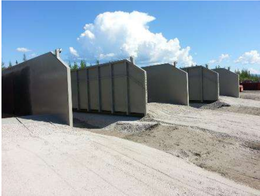
Image E: Soil Containment Facility – 3-sided Bins
