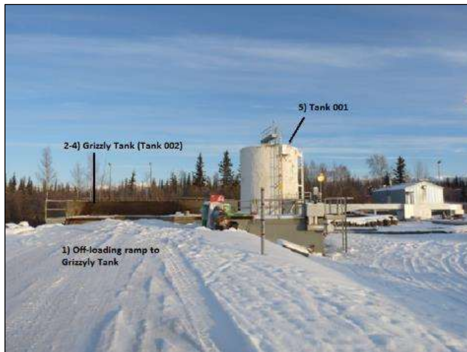
Image F: F-31X Treatment and Injection Facility
