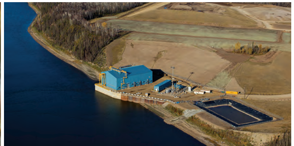
Kearl's water intake facility on the Athabasca River.
