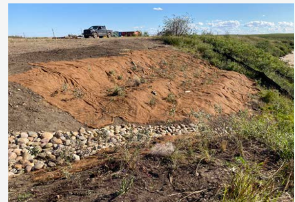
Reclamation activities at our Tuk Base site
