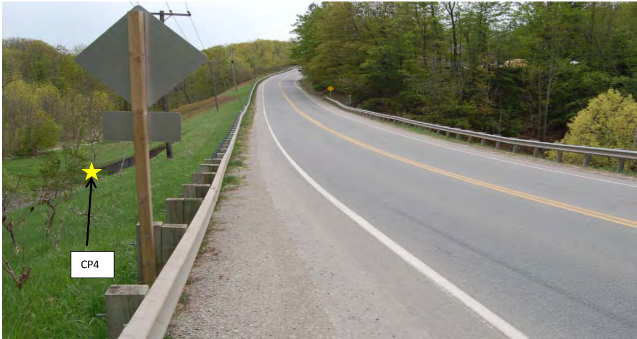
Overview of access to CP4 (Steep embankment– Traffic control required)
