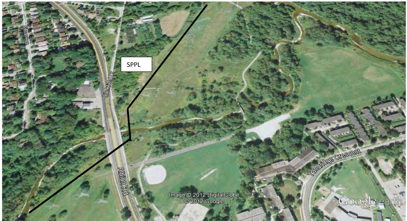
Pipeline River Crossing @ Summerlea Sports Park, 1490 Albion Rd, Etobicoke. (Figure 16C-13)
