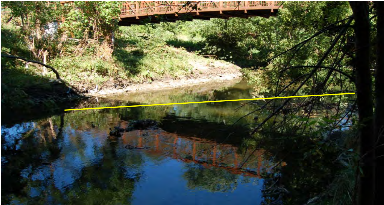
Boom Placement CP2
