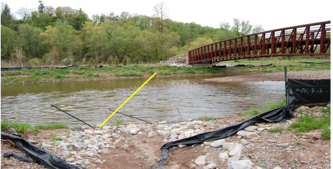
Boom Deployment & Containment CP3
