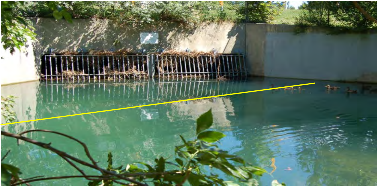
Boom Placement CP4A
