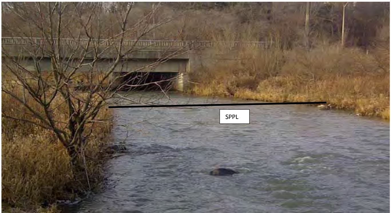
Pipeline Crossing (Figure 16C-2)
