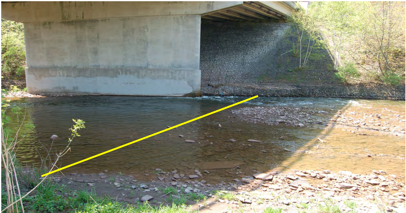
.Boom Deployment & Containment CP2
