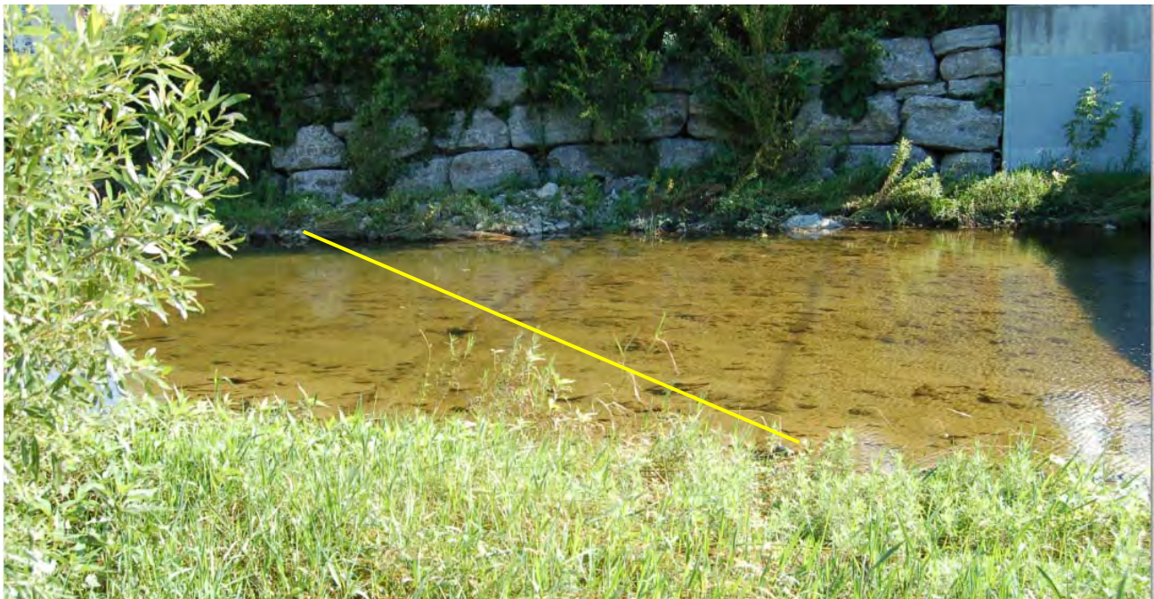
Boom placement CP1
