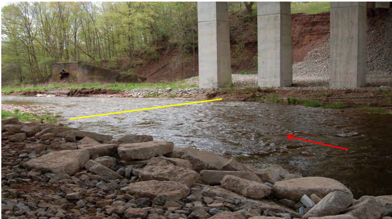
Boom deployment and containment CP2
