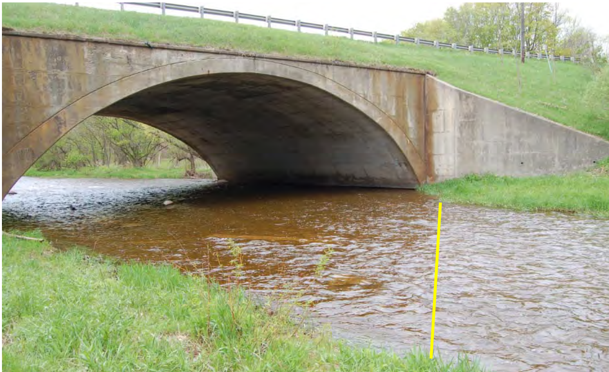
Boom Deployment & Containment CP4
