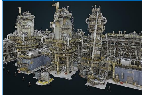
Kearl plant digital twin
