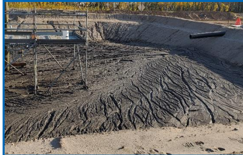
Enhanced in line flocculation
