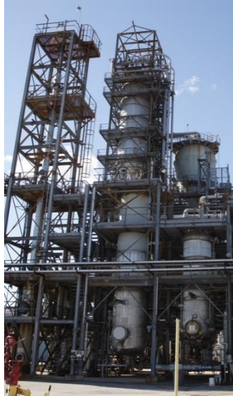
Strategically located refineries
